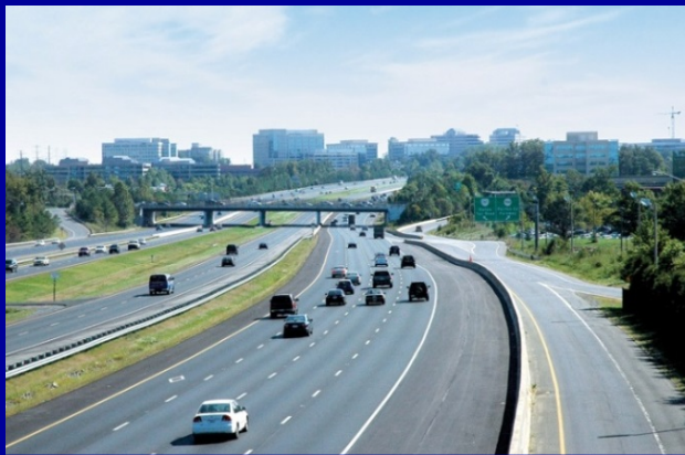
Dulles Toll Road
